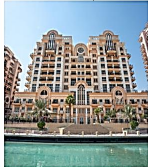
CANAL RESIDANCE PHASE II, UAE
