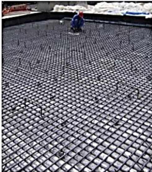
JEBEL ALI WATER RESERVOIRS, UAE
