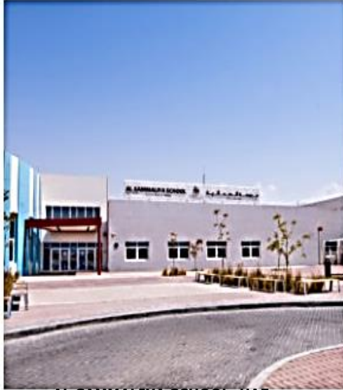
AL SAMMALIYA SCHOOL, UAE
