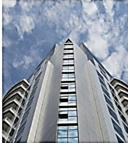
B+G+3P+18 RESIDENTIAL BUILDING, UAE
