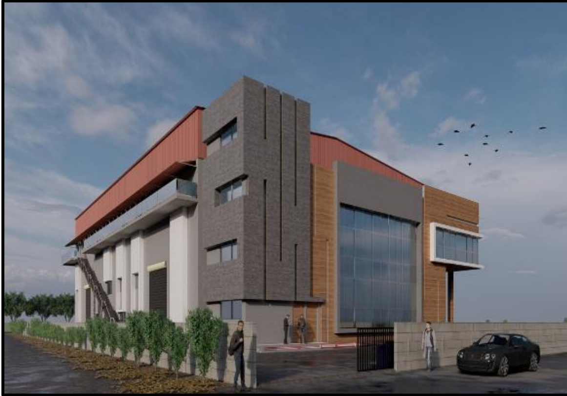
MEHTA PRESSING IV FACILITY IN PUNE
