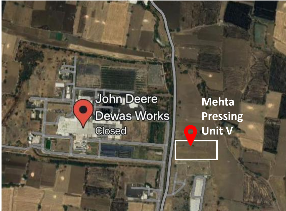
MEHTA PRESSING V FACILITY IN DEWAS
