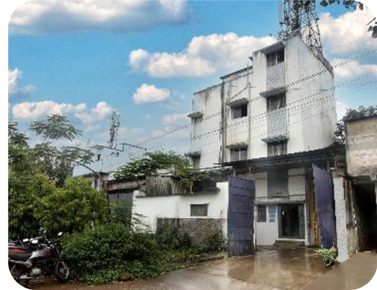
MEHTA PRESSING UNIT-II (MAIN OFFICE)
