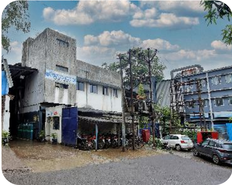
MEHTA PRESSING UNIT I – PUNE (1994)
