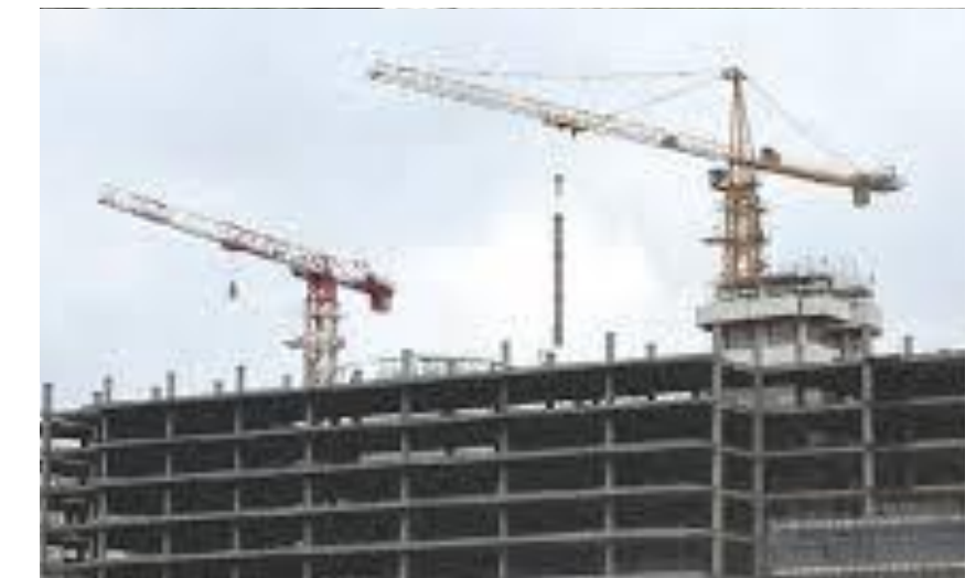
STRUCTURAL STEEL FABRICATION & ERECTION WORK FOR M/S PHOENIX ADVANCE TECHNO PARK, (G+ 18 FLOOR BUILDING) HYDERABAD, (UNDER "KIRBY BUILDING "
