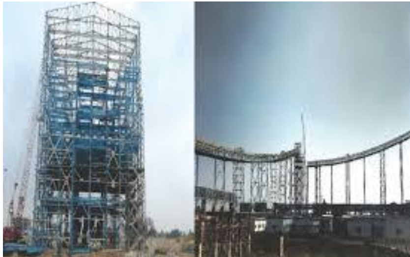
STRUCTURAL STEEL FABRICATION & ERECTION WORK FOR M/S TATA PROJECTS LTD, DARLIPALLI, ORISSA ( NTPC )
