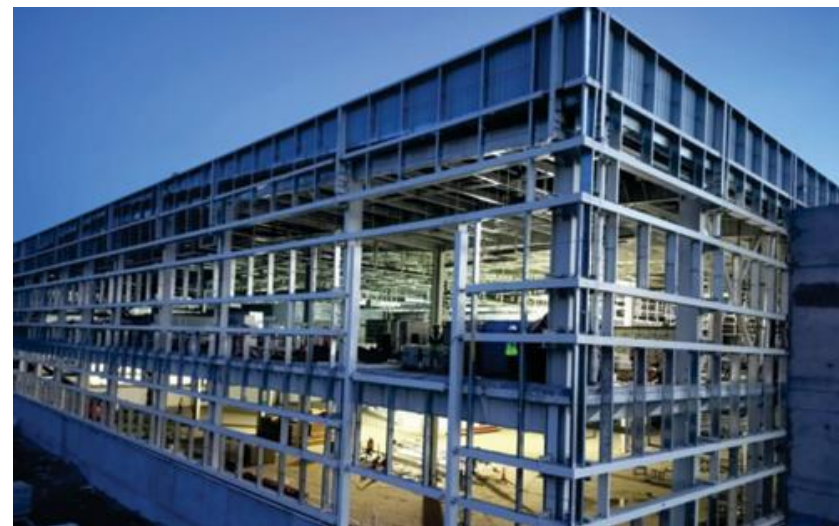
M/S Dr. REDDY'S FORMULATION LTD ( STRUCTURAL STEEL DESIGN & DETAIL ENGINEERING, MANUFACTURING, SUPPLY AND ERECTION OF PRODUCTION BUILDING)
