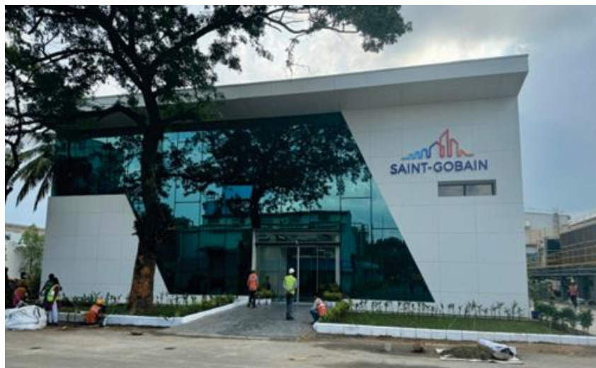
M/S SAINT GOBAIN INDIA PVT LTD ( STRUCTURAL STEEL DESIGN & DETAIL ENGINEERING, MANUFACTURING, SUPPLY AND ERECTION OF OFFICE CUM CANTEEN BUILDING - GREEN BUILDING )
