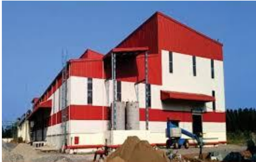
M/S PIDILITE INDUSTRIES LTD (STRUCTURAL STEEL DESIGN & DETAIL ENGINEERING, MANUFACTURING AND ERECTION OF CC AGGREGATE BUILDING )
