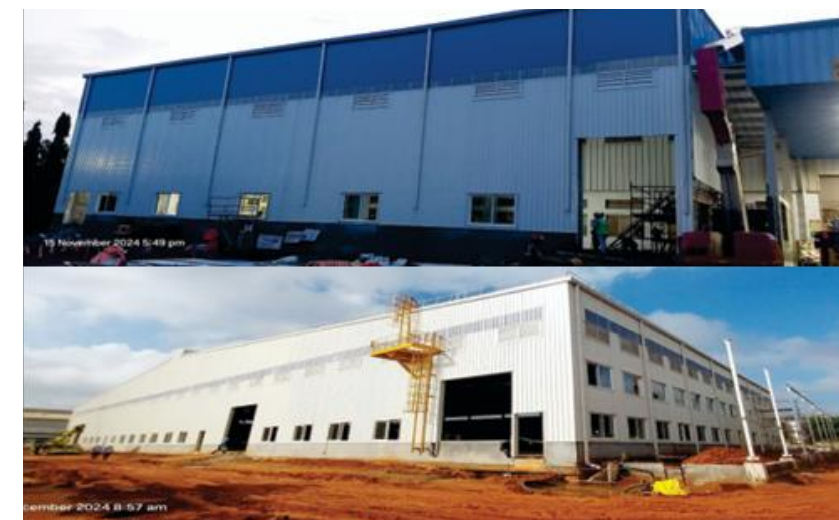
M/S SAINT GOBAIN INDIA PVT LTD - WEBER ( STRUCTURAL STEEL DESIGN & DETAIL ENGINEERING, MANUFACTURING, SUPPLY AND ERECTION OF PU & SEALANT MANUFACTURING BUILDING )
