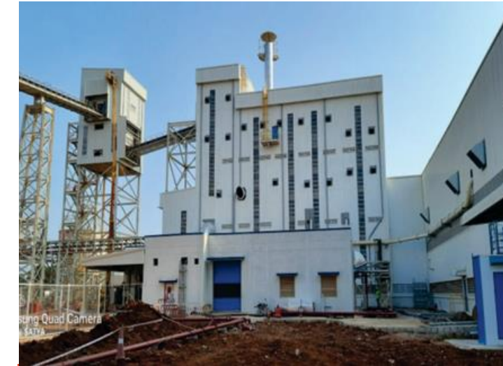
M/S SAINT GOBAIN INDIA PVT LTD, VISAKHAPATNAMA. (STRUCTURAL STEEL DESIGN & DETAIL ENGINEERING, MANUFACTRING, ERECTION & EQUIPMENT INSTALLATION WORK FOR MILL BUILDING)
