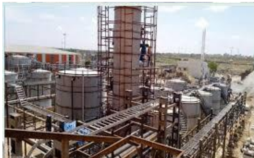
DETAIL ENGINEERING, FABRICATION AND ERECTION OF PROCESS TANK FOR M/s WIPRO PERSONAL AND HOME CARE
