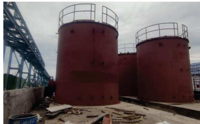
DETAIL ENGINEERING, FABRICATION AND ERECTION OF 80KL TANK FOR M/s ATC TIRES PRIVATE LIMITED
