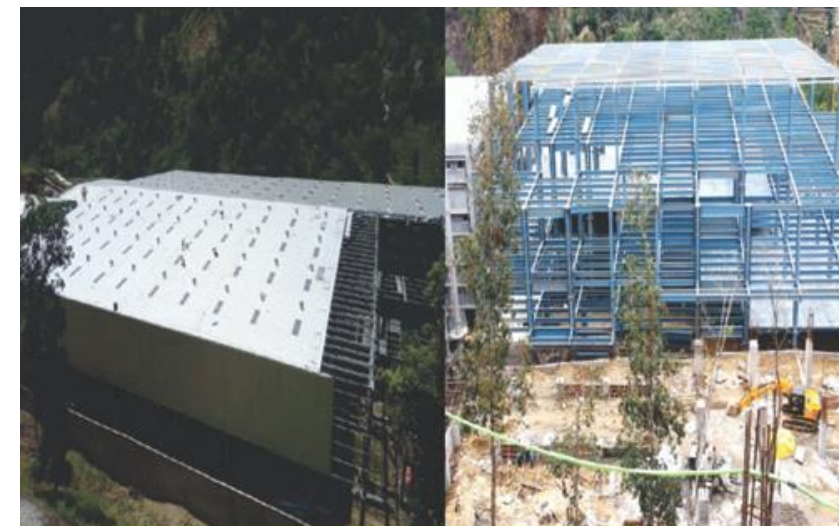
INSTALLATION OF PRE-ENGINEERING BUILDING OF PHARMA STRUCTURAL FOR MIS MANKIND PHARMALTD
