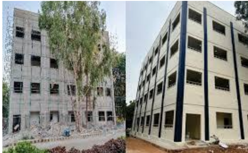
THE ICFEI FOUNDATION FOR HIGHER EDUCATION ( CIVIL, MEP & STRUCTURAL STEEL DESIGN & DETAIL ENGINEERING, MANUFACTURING SUPPLY AND ERECTION OF FST CLASS ROOM, (TURNKEY PROJECT) )
