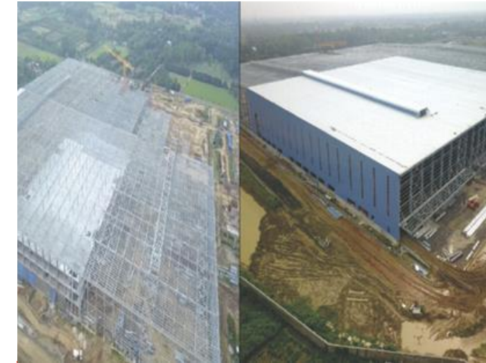
INSTALLATION OF PREENGINEERING FOR M/S INSTAKART SERVICES PVT LTD, WEST BENGAL
