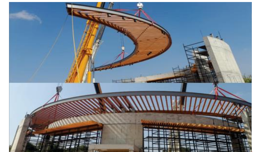
M/S AUROBINDO REALTY & INFRASTRUCTURE PVT LTD (STRUCTURAL STEEL DESIGN & DETAIL ENGINEERING, MANUFACTURING, SUPPLY AND ERECTION OF ENTRY GATE PORTAL )
