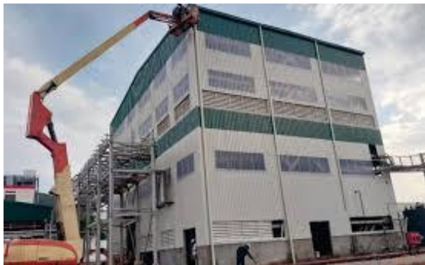
M/S GRANULES CZRO PVT LTD (STRUCTURAL STEEL DESIGN & DETAIL ENGINEERING, MANUFACTURING, SUPPLY AND ERECTION OF PRODUCTION BUILDING)
