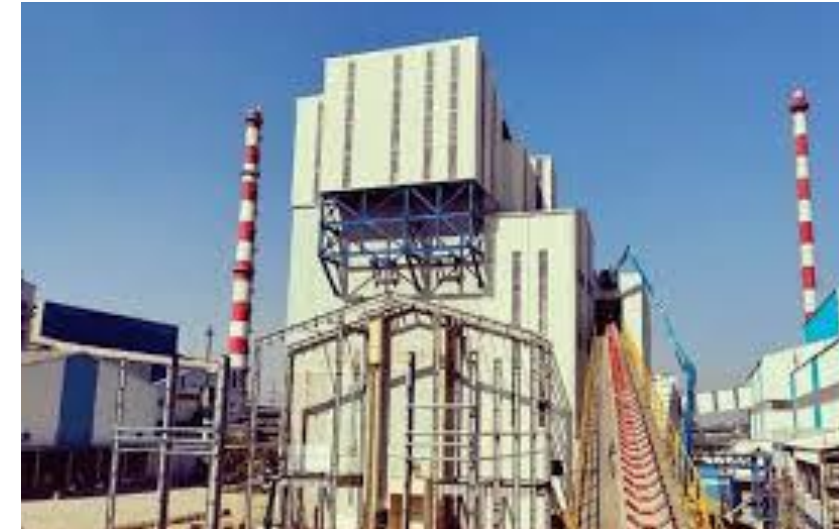
M/S SAINT GOBAIN INDIA PVT LTD, BHIWADI, RAJASTHAN ( STRUCTURAL STEEL DESIGN & DETAIL ENGINEERING, MANUFACTURING, SUPPLY AND ERECTION OF CULLET HEAD HOUSE BUILDING )
