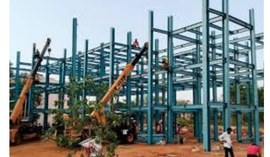
THE ICFEI FOUNDATION FOR HIGHER EDUCATION ( CIVIL, MEP & STRUCTURAL STEEL DESIGN & DETAIL ENGINEERING, MANUFACTURING, SUPPLY AND ERECTION OF HOSTEL B-BLOCK, (TURNKEY PROJECT) )
