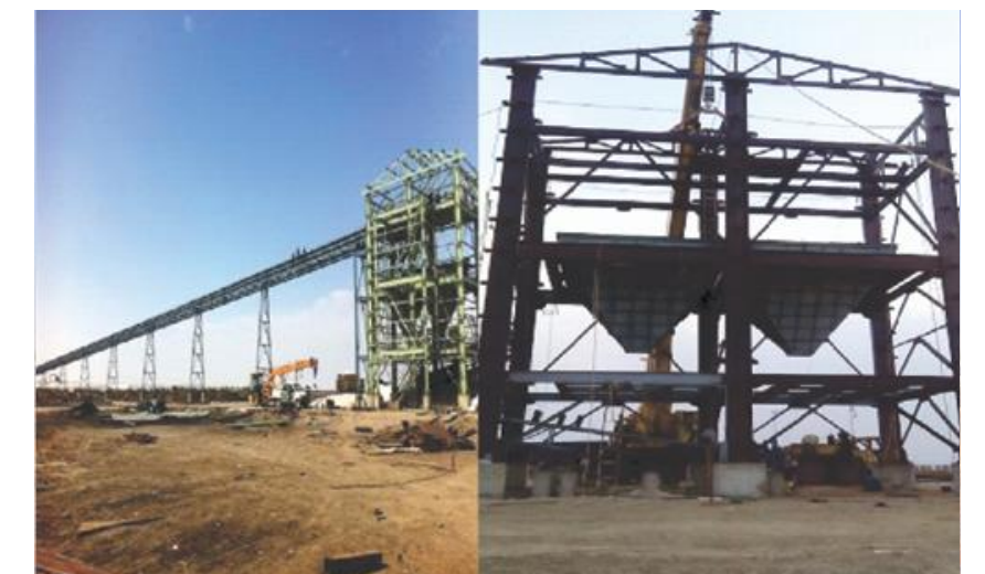
DESIGN, MANUFACTURING, SUPPLY AND ERECTION OF 350 MTR 800 MM BELT WIDTH CONVEYOR FOR ARCHEAN CHEMICALS
