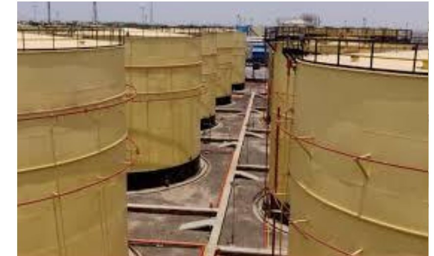
DETAIL ENGINEERING, FABRICATION & ERECTION OF TANK FOR PETROLIUM PRODUCTS M/S SHREEJI LIQUID STORAGE TERMINALS PVT LTD, KANDLA PORT, GANDHIDHAM, GUJARAT
