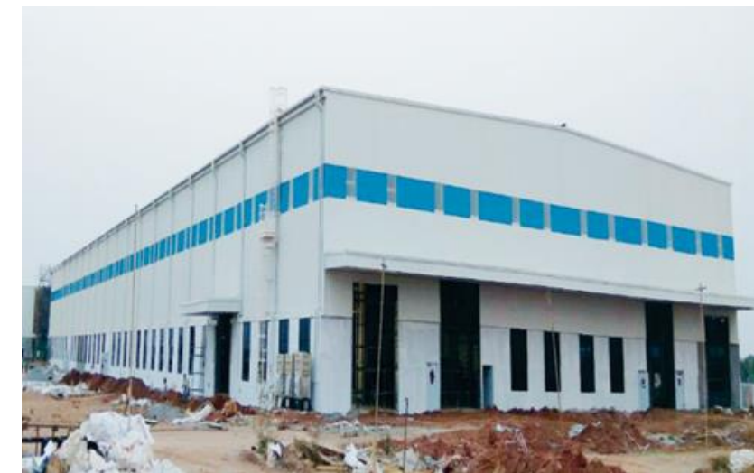
INSTALLATION OF PRE-ENGINEERING BUILDING MIS TATA BOEING AEROSPACE LIMITED, HYDERABAD
