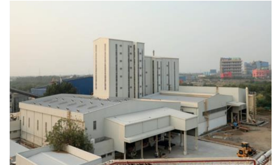
M/S SAINT GOBAIN INDIA PVT LTD, JHAGADIA, GUJARAT ( STRUCTURAL STEEL DESIGN & DETAIL ENGINEERING, MANUFACTURING, SUPPLY AND ERECTION OF FG & GYPSUM BUILDING )
