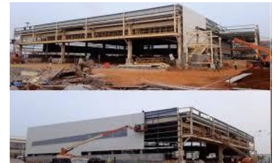
M/S SAINT GOBAIN INDUSTRIES INDIA LTD (STRUCTURAL STEEL DESIGN & DETAIL ENGINEERING, MANUFACTURING, SUPPLY AND ERECTION OF WAREHOUSE BUILDING )
