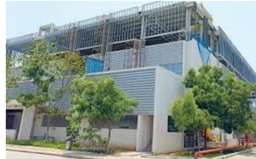
M/S Dr. REDDY'S LABORATORIES LTD ( STRUCTURAL STEEL DESIGN & DETAIL ENGINEERING, MANUFACTURING, SUPPLY AND ERECTION OF HARMONE BUILDING)
