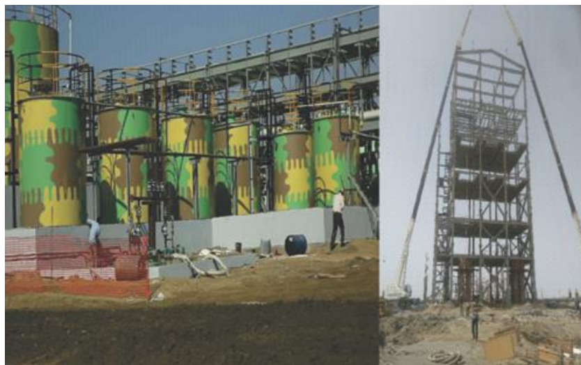
DESIGN ENGINEERING, FABRICATION & ERECTION OF BROMINE PLANT & BROMINE TANK FOR MIS SATYESH BRINCHEM PVT LTD, GUJARAT
