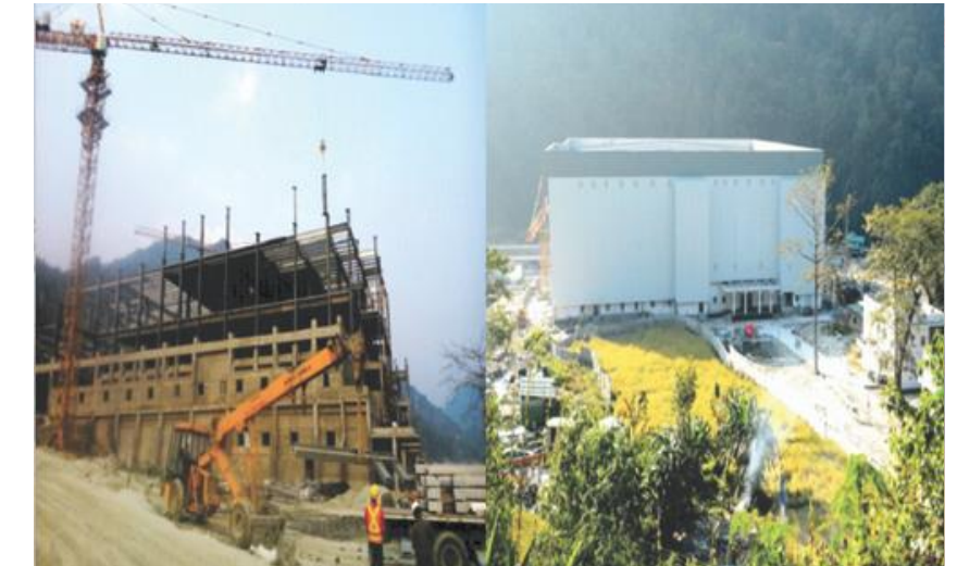
INSTALLATION OF PRE-ENGINEERING BUILDING FOR CIPLA LTD
