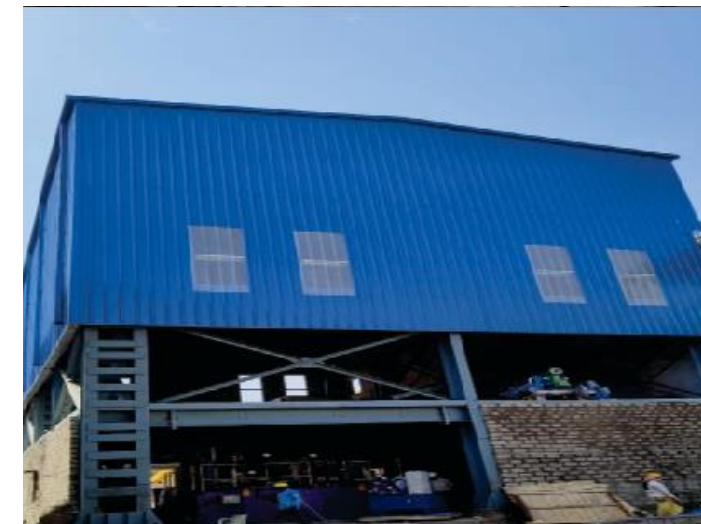
M/S LAURUS LABS LIMITED, VISAKHAPATNAMA. (STRUCTURAL STEEL DESIGN & DETAIL ENGINEERING, MANUFACTRING, ERECTION & EQUIPMENT INSTALLATION WORK FOR TG BUILDING)
