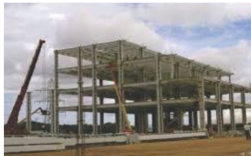
PROCESS PLANT STRUCTURE, EQUIPMENT AND PIPING ERECTION FOR BASF
