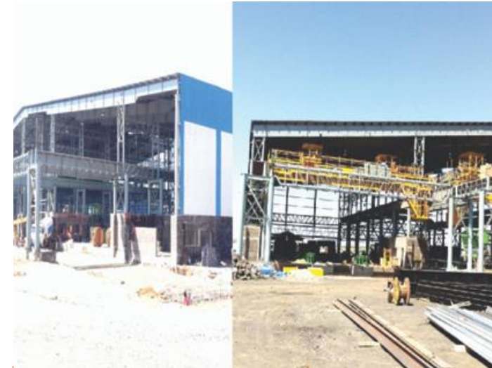
M/S WELSPUN WASCO PVT [TO, AWH. STRUCTURAL STEEL DESIGN & DETAIL ENGINEERING, MANUFACTURING OF PRE ENGINEERING BJIUNDG. INSTALLATION WORX EQUIPMENT I
