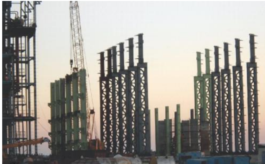
DETAIL ENGINEERING, FABRICATION AND ERECTION OF TG BUILDING STRUCTURE FOR ARCHEAN CHEMICALS
