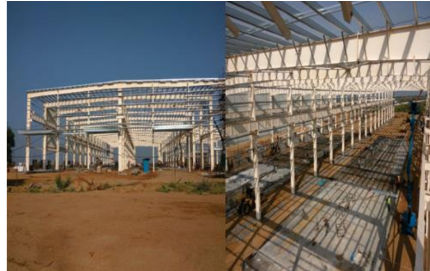
M/S TATA ADVANCED SYSTEMS LIMITED. ( STRUCTURAL STEEL DESIGN & DETAIL ENGINEERING, MANUFACTURING OF PRE ENGINEERING BUILDING, INSTALLATION WORK & EQUIPMENT ERECTION )
