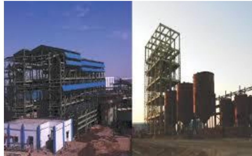
DETAIL ENGINEERING, FABRICATION AND ERECTION OF PLANT STRUCTURE PIPE RACKS , PIPING AND TANK FARMS FOR ARCHEAN CHEMICALS
