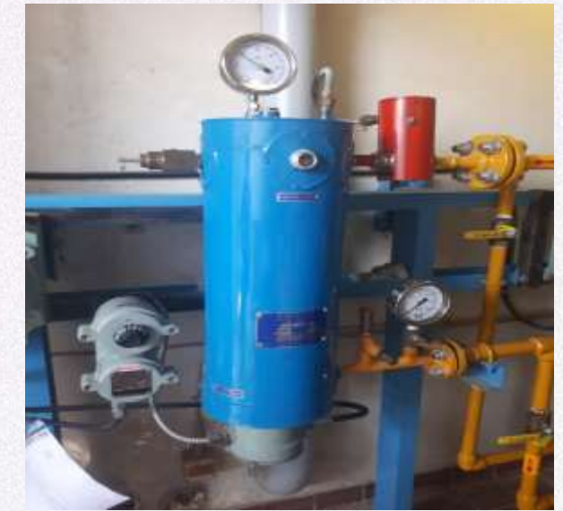
Vaporizer Installation
