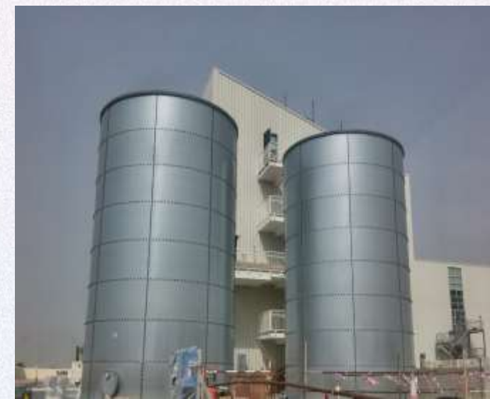
API 650 Site Erected Storage Tank
