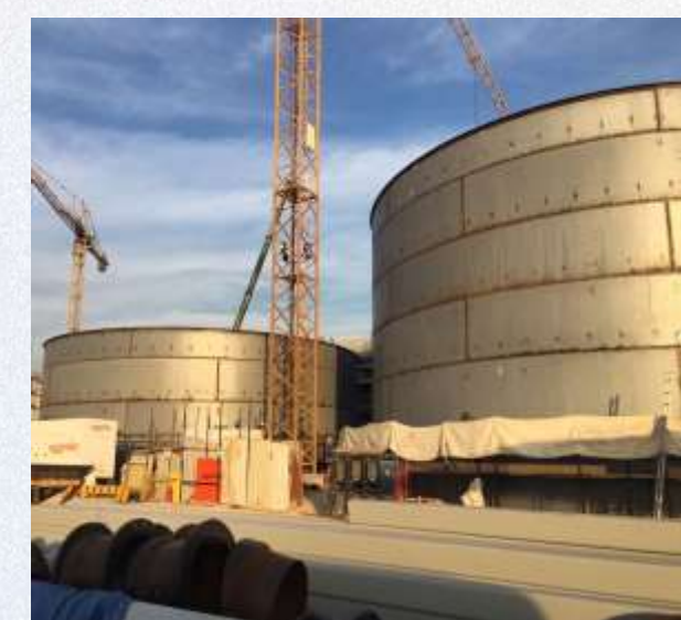
750M3 API 650 Site Erected Tank
